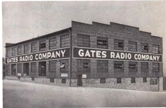
Gates warehouse and regular shipping point. It is one of the most strategically located buildings in Quincy in relation to air, rail and truck shipping.
