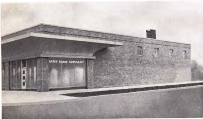
Houston, Texas, stock carrying branch located at 2700 Polk Avenue, telephone Capitol 8-8536.
